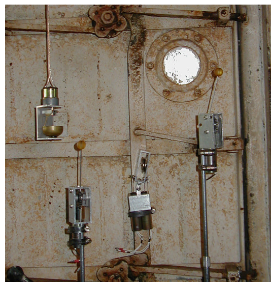
Figure 5: Several ModBots in installation
